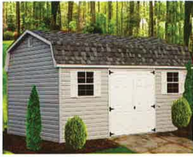
Dutch Barn with vinyl siding
